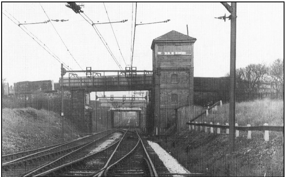
Crowthorn Junction signal box c1954 looking north. The Woodhead electrification included this section of the OA&GB as far as Ashton Moss South exchange sidings. The first bridge, Crowthorn Lane has been raised temporarily, while the second bridge, Ashton Old Road, has already been rebuilt. The bridges made the observation of trains approaching from the north difficult.
